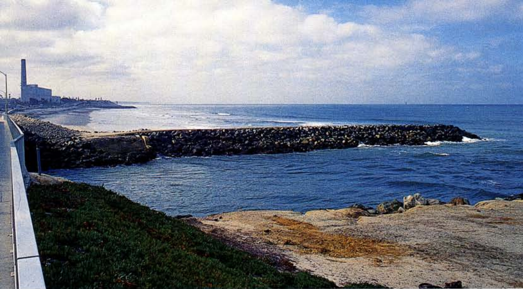
Carlsbad city beaches represent a supreme effort by state and local agencies to prevent further loss of recreational seaside property. Jetties have been constructed (left), while acres of sand have been pumped in and distributed on the beach (below and bottom) to replace that lost to erosion.
