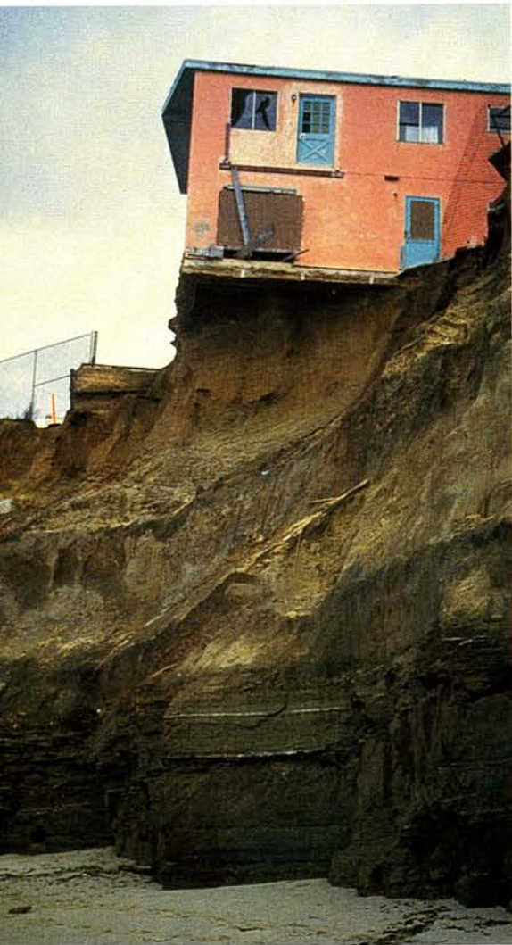
Storm-driven coastal erosion imperils seaside development in San Diego County.
