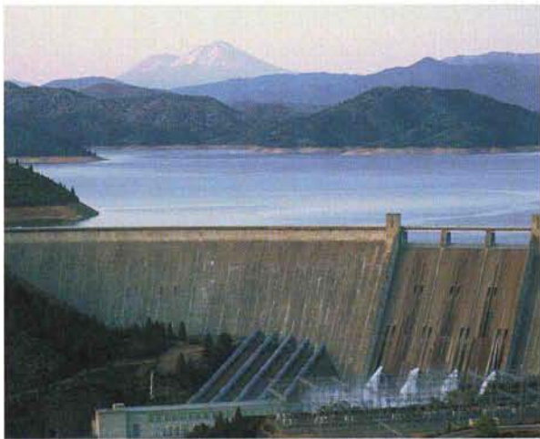
Above, Shasta Dam in northern California.
