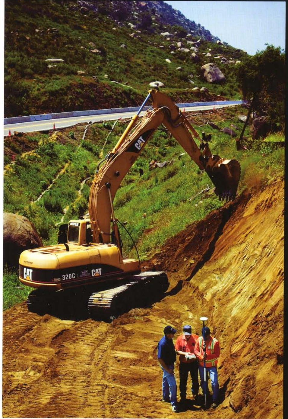
Yehuda Bock (left) and San Diego County surveyors assessed GPS readings of a road-widening project off Wildcat Canyon Road south of the Barona Indian Reservation.
