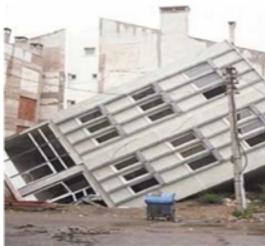
Liquefaction
